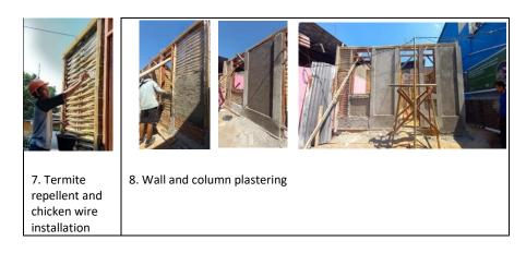
**Figure 3** Plastered-bamboo construction stages. Image Copyright, Authors (2023)
