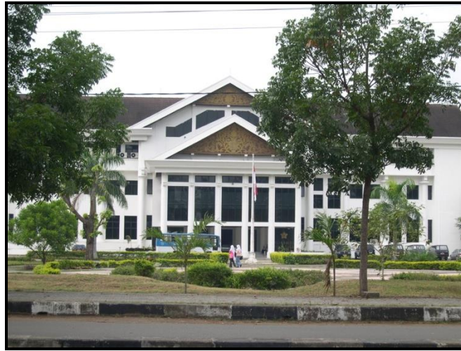
Figure 4 Directorate building, University of Syiah Kuala, built-in 1990s with the reference of traditional Source: Author's collection
