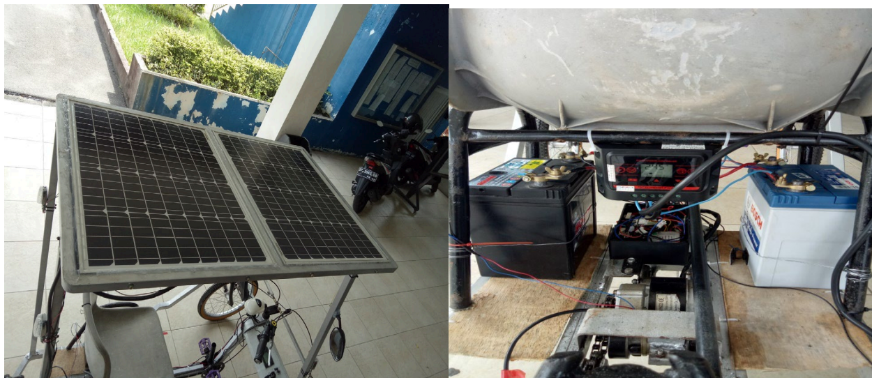
Figure 2. Solar panel and control system
