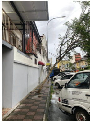
Figure 3. Show Lack of Maintenance
