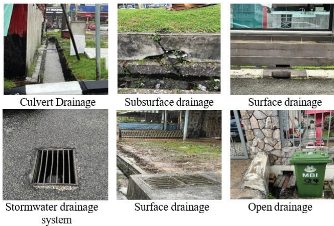
Figure 2. Type of Drainage at Taman Fair Park Ipoh, Perak
