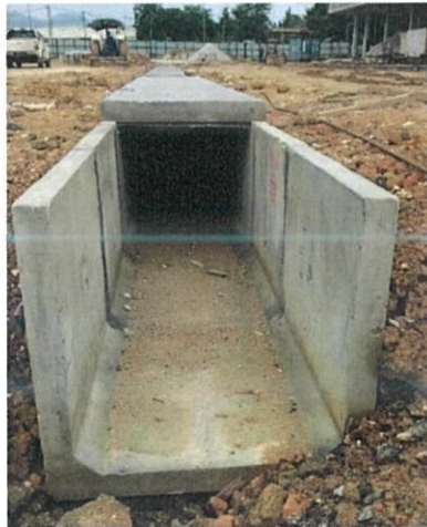
Figure 1.1: Under construction drain.
