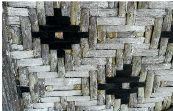
Figure 6 : Current condition of the kelarai walls of Ihsaniah Iskandariah Mosque, Padang Rengas. (Source: Syed Abdul Haris et. al., 2024)
