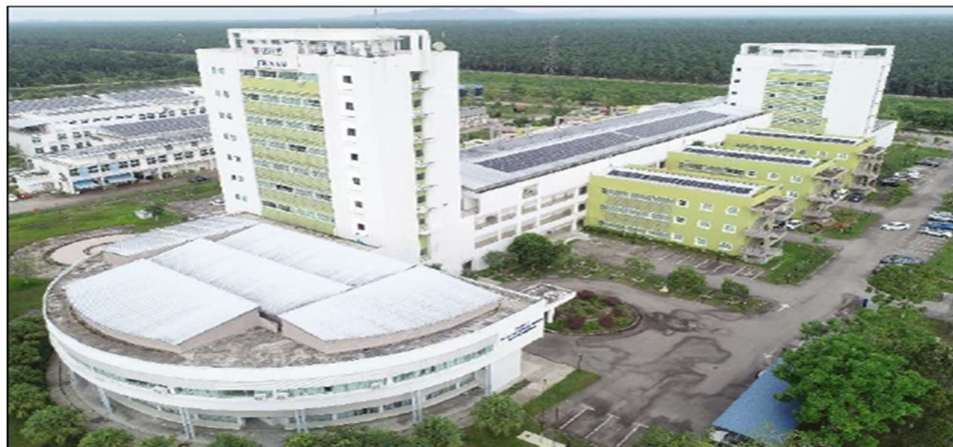
Figure 1. The installation of panel solar at FKAAB UTHM.
