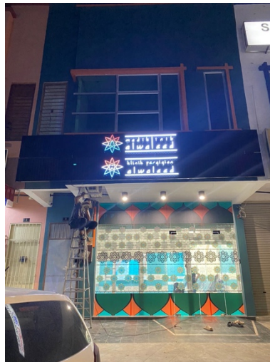
Figure 12: The image of clinic entrance during construction
