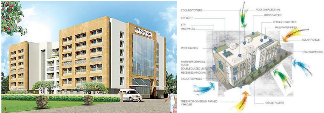
Figure 6: Kohinoor Hospital in Kurla, India (inspiration)
