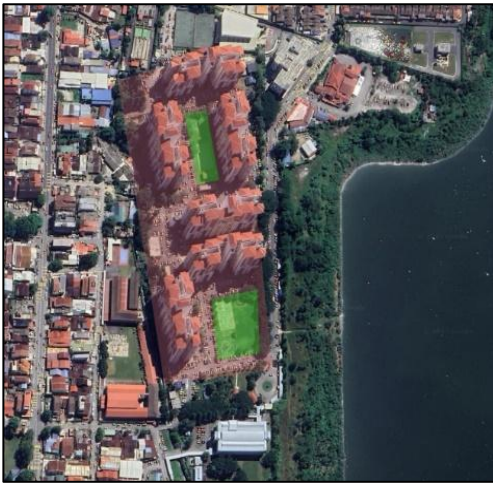
Fig. 3. Aerial view of PPR Beringin
