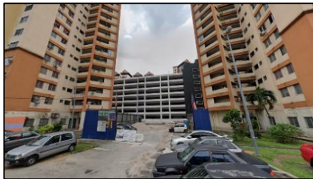
Fig. 9. After Construction of Podium Parking
