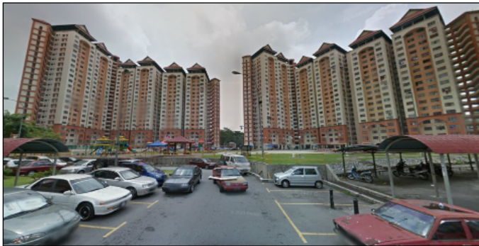
Fig. 10. Before construction of podium parking
