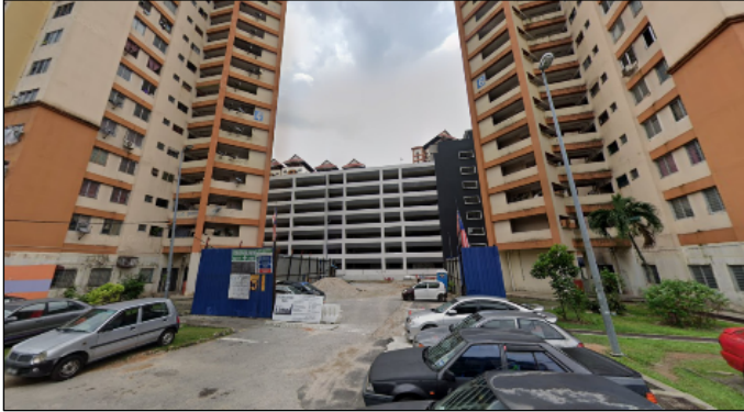
Fig. 11. After construction of podium parking
