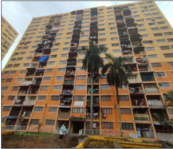
Fig. 3. Flat External Courtyard Lacks Natural Environment Element.
