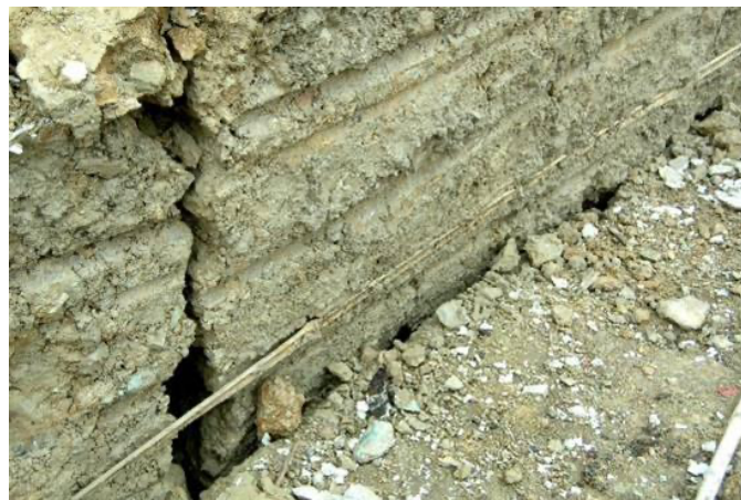
Fig. 8. Rammed Earth Wall
