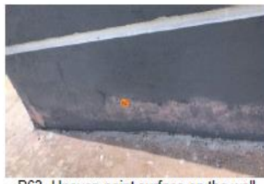
P63- Uneven paint surface on the wall
