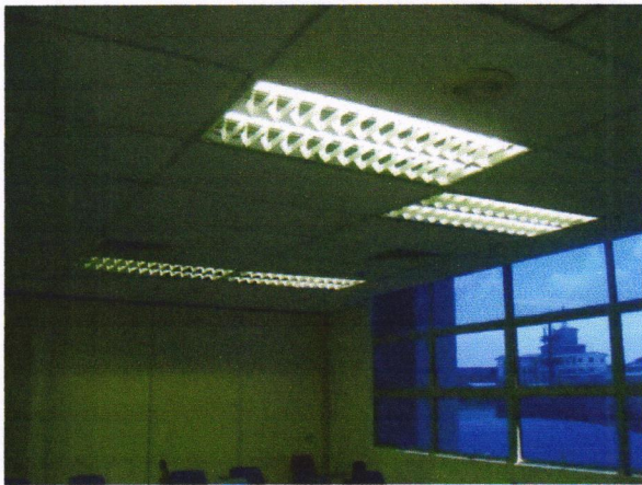
Figure 2.3: Arrangement of lighting system at lecture room
