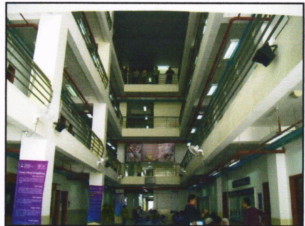
Figure 2.1: The lighting system at the corridor daytime
