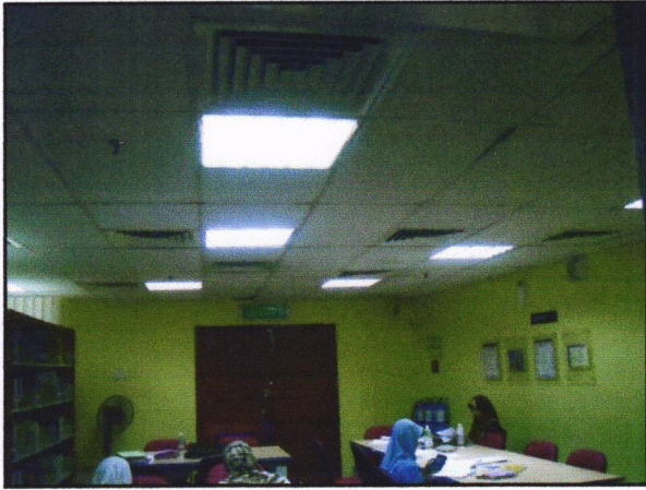
Figure 2.2: Type of lamp that use at PTAR 3
