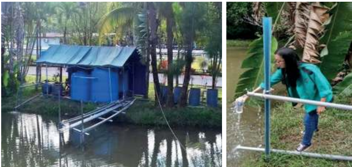
Figure 5.10 Water Treatment Pilot Plant At The Pond In Samarahan Campus
