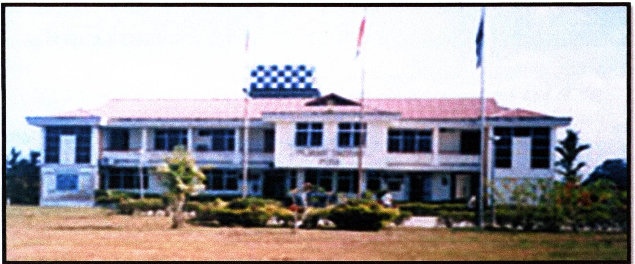
Figure 1: Pusa Sub-district Office
