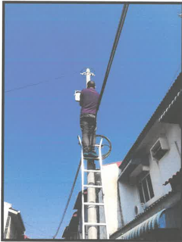
Figure 3.1.6(a) : Installation of fiber cable from the DP to the building
