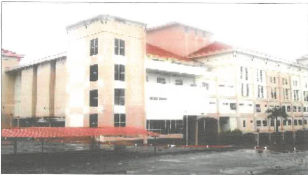
Figure 4: ACC (Ambulatory Care Centre) Building
