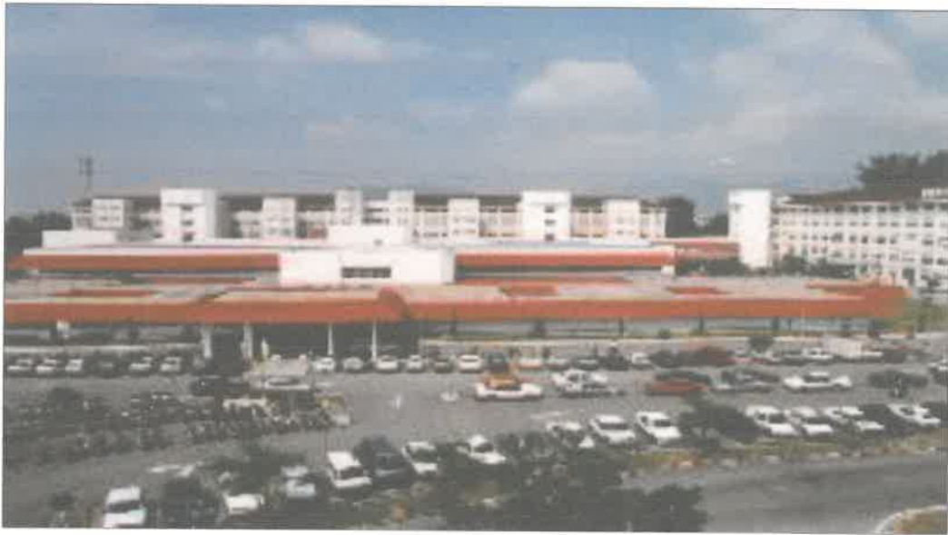
Figure 3: Current view of HPP
