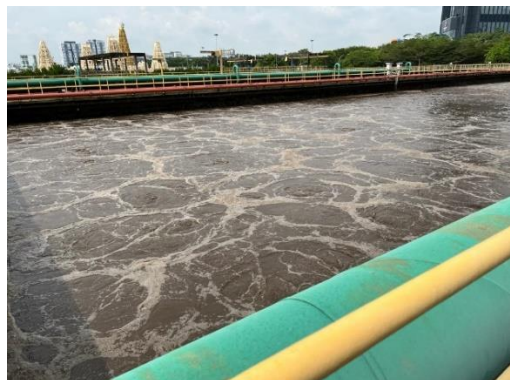
Figure 1: Wastewater from aeration tank in IWK
