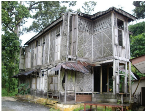
Figure 1. The Condition of the Mosque after being Vacated in 1976
