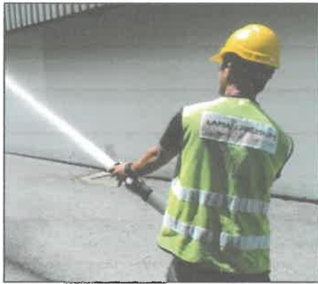
Figure 3.46: Water pressure checking.
