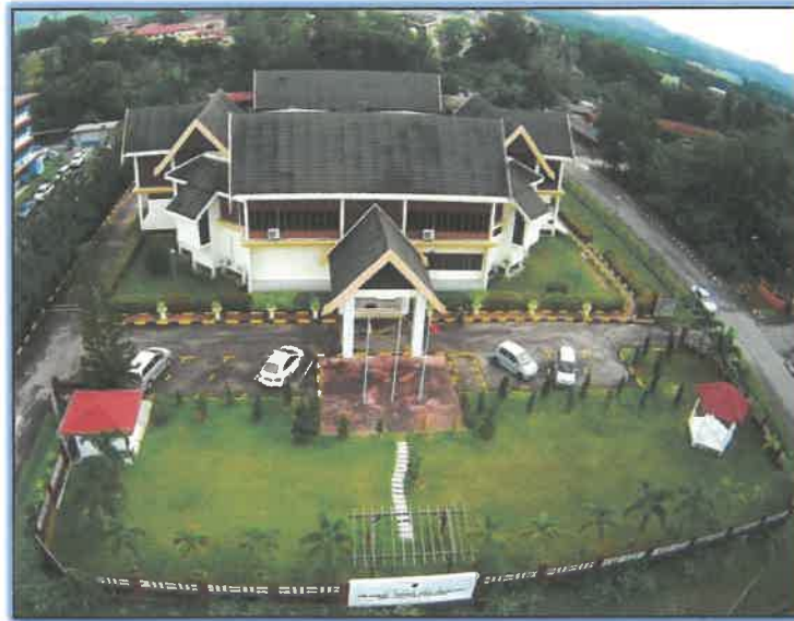
Figure 1.2: Department of Land and District of Kuala Krai Building
