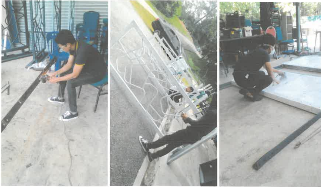
Figure 6: Shows trainee doing work progress during 3R project
