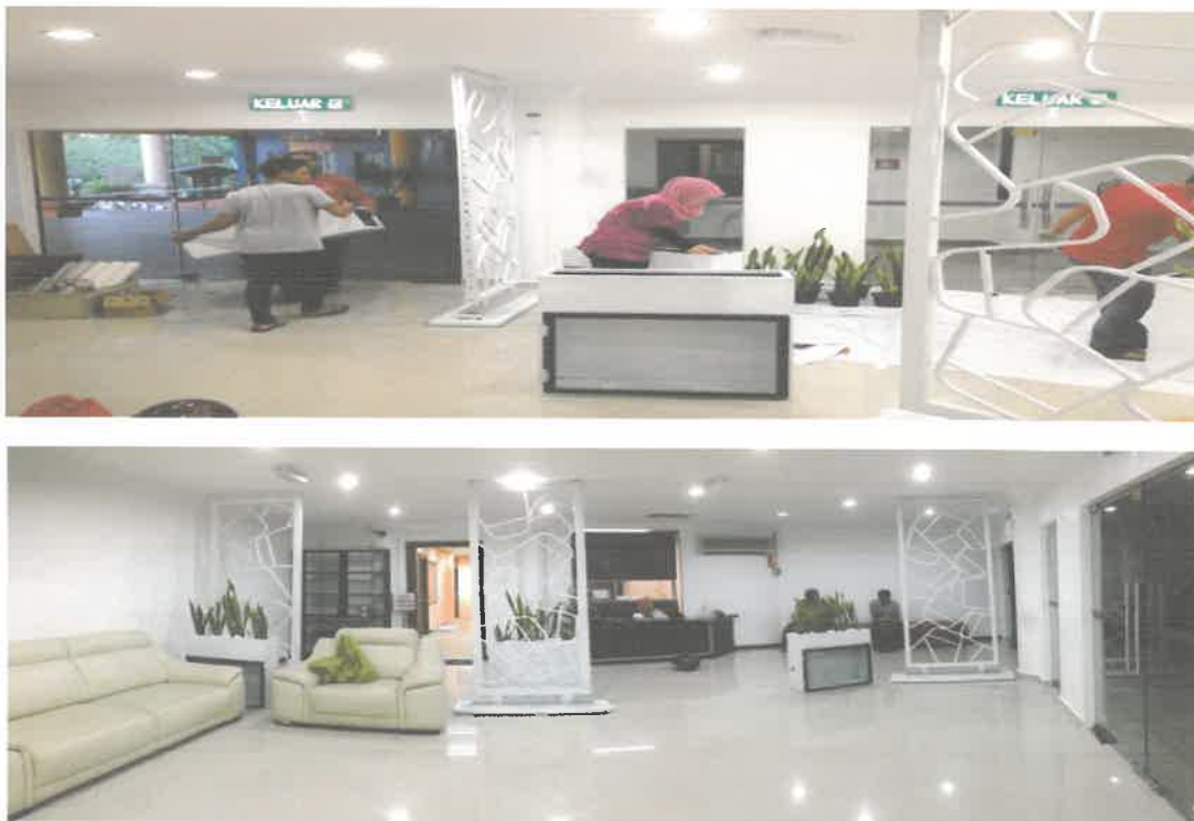
Figure 7: Shows trainee doing the installation and finishing process of the project
