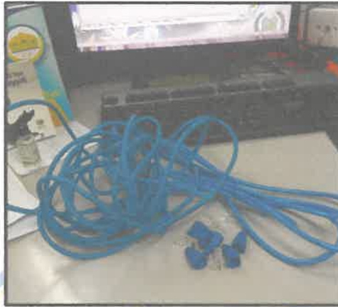
Figure 3.4: Network cabling activity
