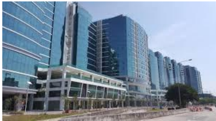
Figure 4: UOA Business Park
