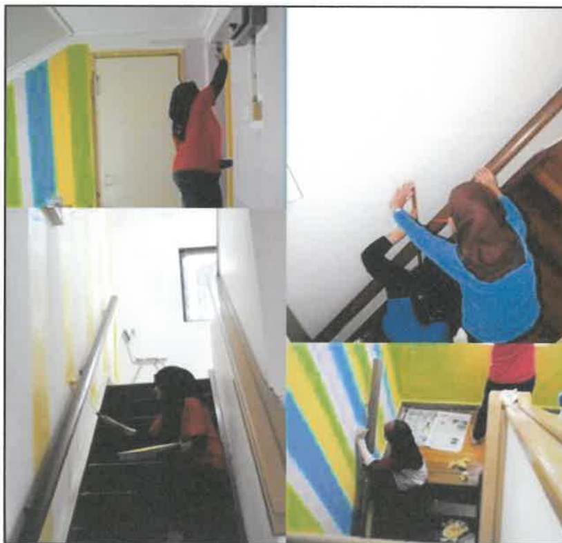
Figure 3-28: Measure and Paint the Stairways
