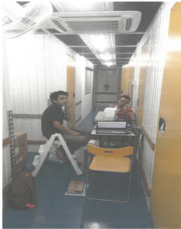
Figure 23: Physical Check & DAMS Test
