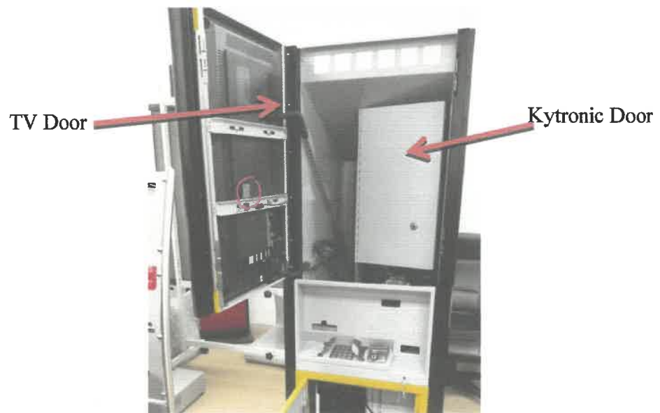
Figure 27: Zone A Kiosk Door
