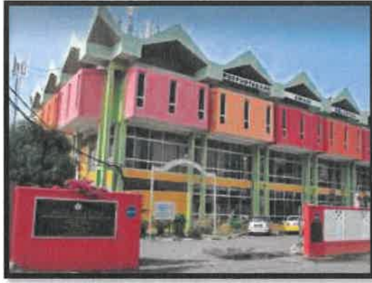
Figures 2.2: Building of Perbadanan Perpustakaan Awam Kelantan
