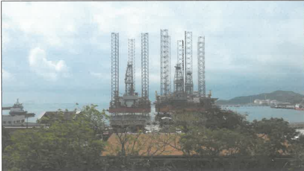
Figure 36: Platform of Epic Company
