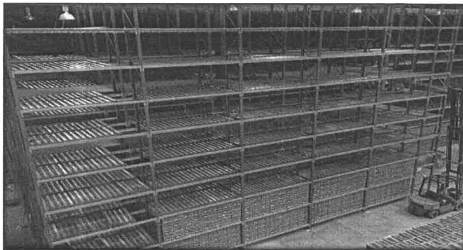
Figure 3: Rack In Warehouse
