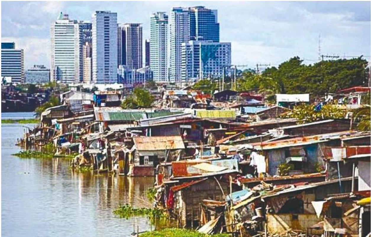
Picture 1: Illegal houses built in the city center.
