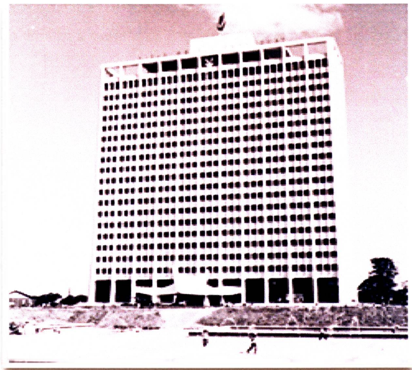
Figure 1.3 Wisma Bapa Malaysia Building
