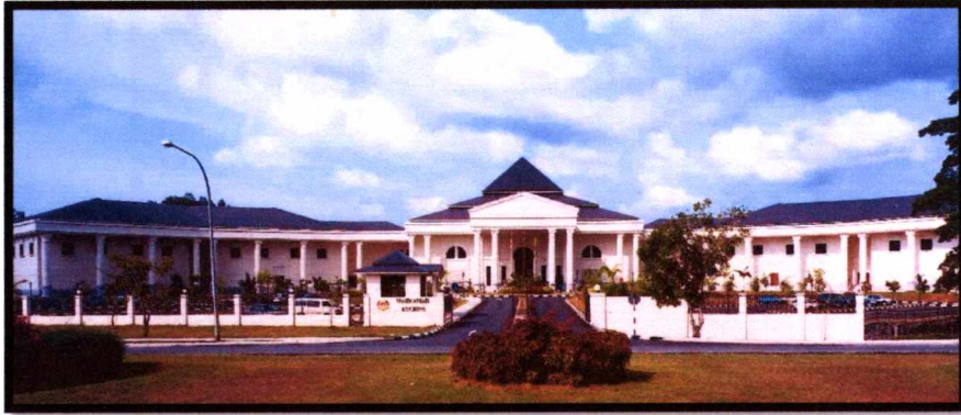
Kuching High Court Complex
