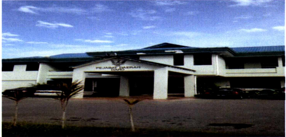
Figure 1: Daro District Office
