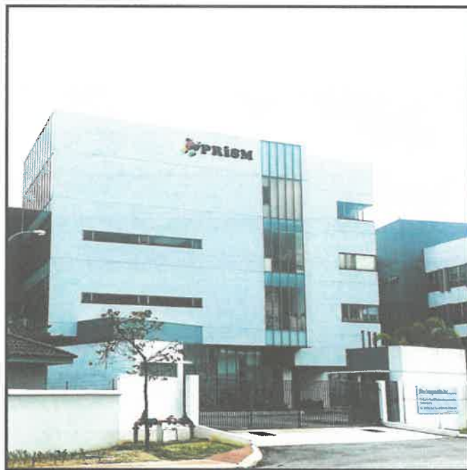
Figure 1.1: Entrance of main building Prism Integrated Sdn Bhd
