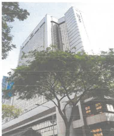
Figure 1: The EPF Head Office building
