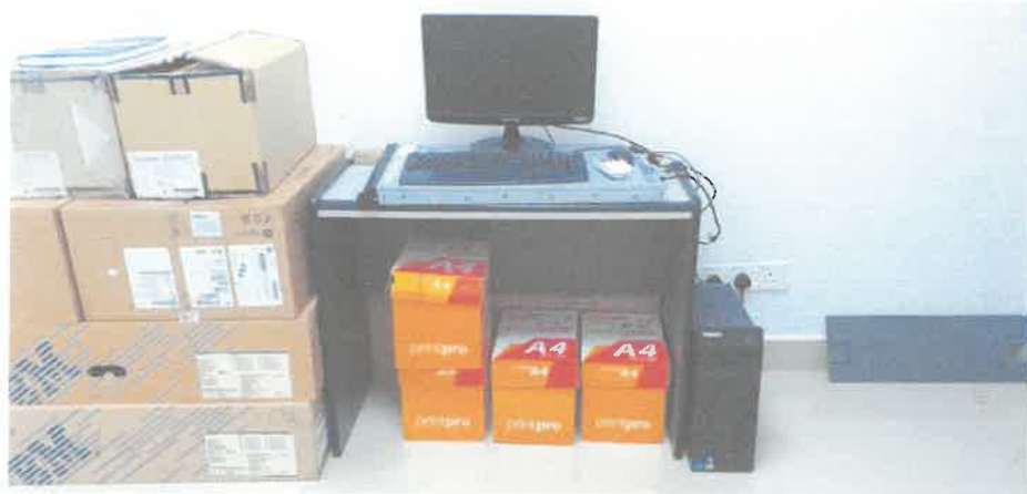
Figure 11 ; The hardware that have been clean up at the server room
