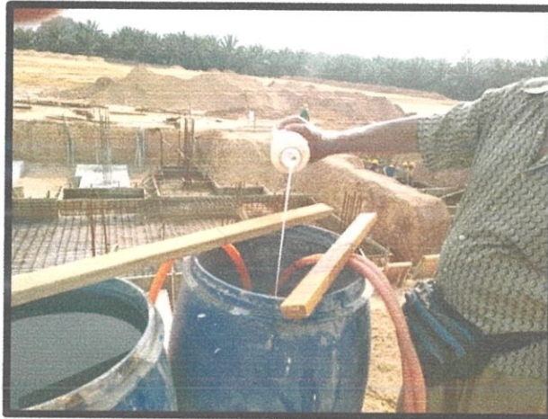
Figure 3.13 The anti-termite mix with the water
