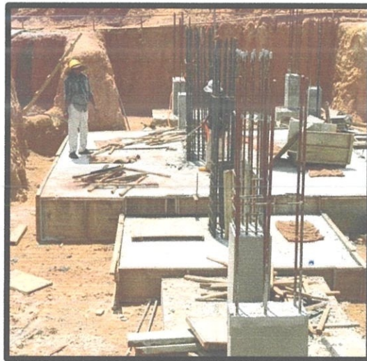
Figure 3.25 Dismantle the formwork of column stump
