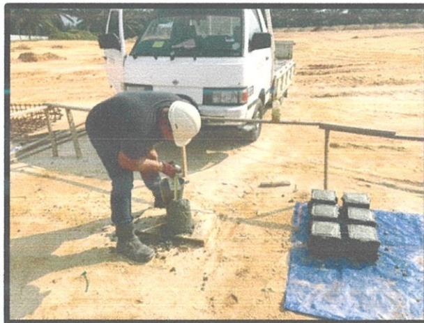
Figure 3.21 Slump 85mm and cube on site
