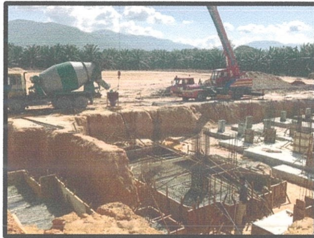
Figure 3.22 Concrete works for pad foundation.
