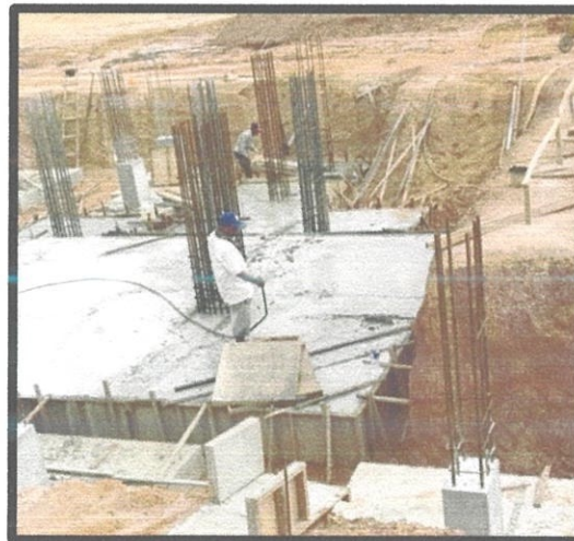
Figure 3.27 The curing process
