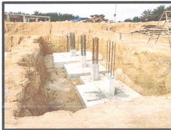
Figure 3.2 Pad foundation
