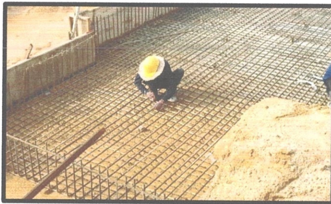
Figure 3.19 The workers tie the reinforcement bar
