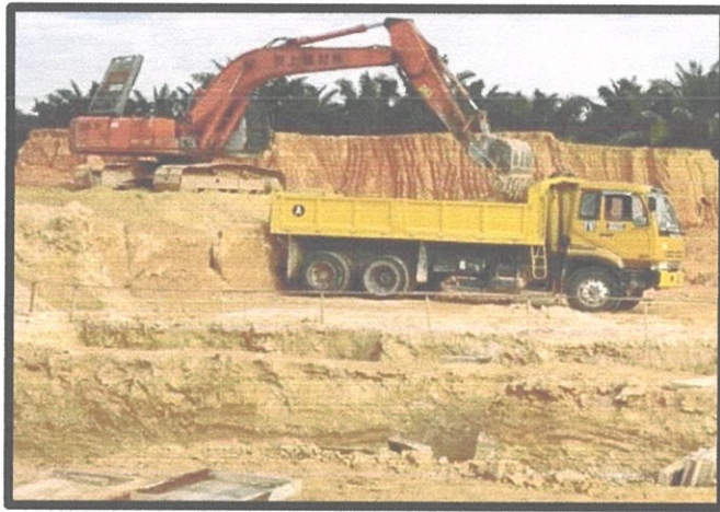
Figure 3.8 Placed the soil in the dumpy truck
