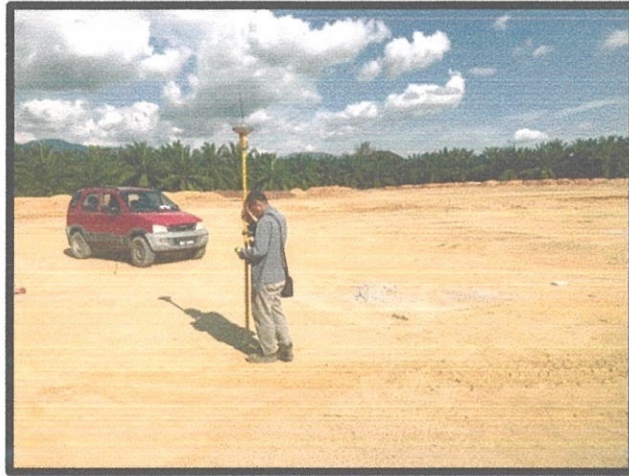
Figure 3.5 The surveyor setting out the tools
