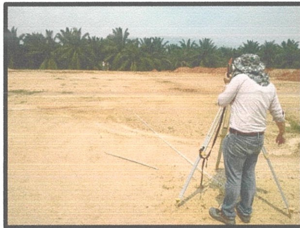
Figure 3.4 Setting out work
