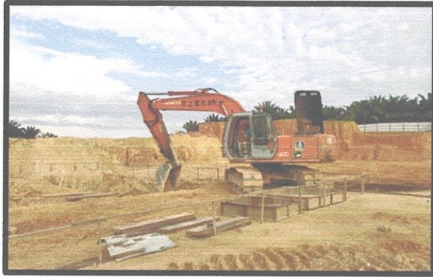
Figure 3.7 The excavators dig the hole for pad foundation
