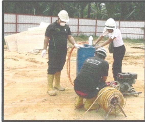
Figure 3.15 Using water jet to spread the anti-termite
