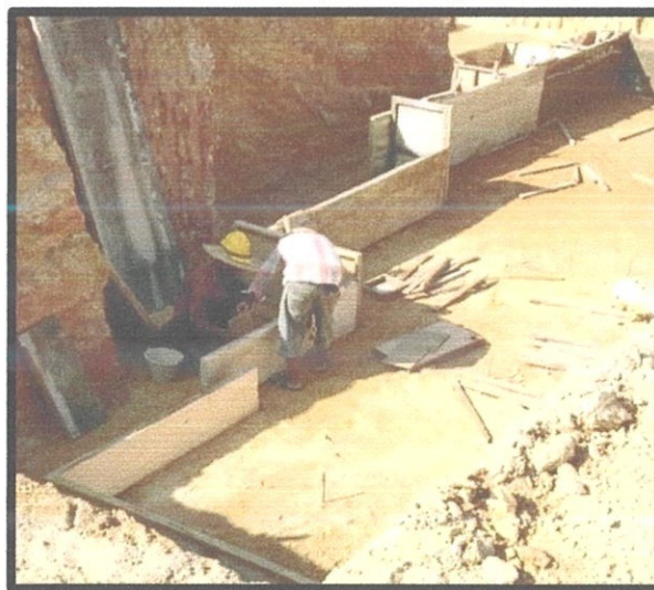
Figure 3.12 The workers install the formwork of pad foundation
