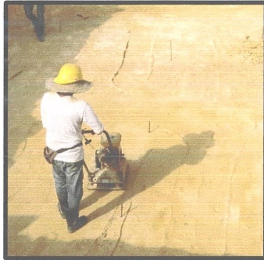
Figure 3.9 Compact the soil
