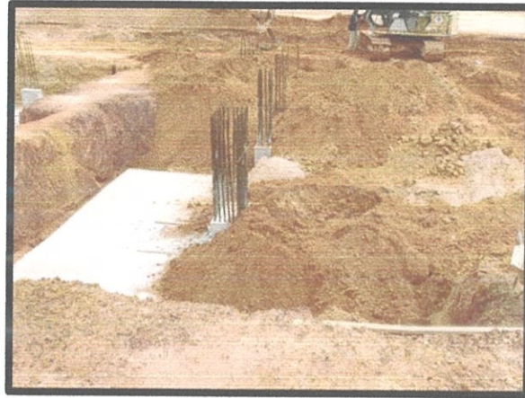
Figure 3.28 Backfill to the pad foundation
