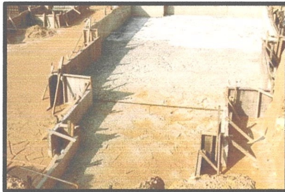
Figure 3.16 Lean concrete to pad foundation
