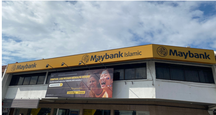
Figure 1: Maybank Ipoh Garden Branch Building
