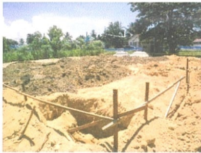
Figure 9 shows the excavation process.
