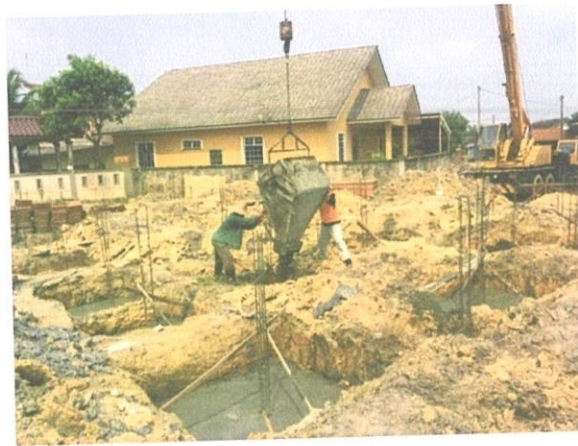
Figure 13 shows the process of pour the concrete using a bucket crane.
