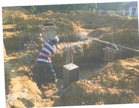
Figure 15 shows the process of dismantle the formwork.
