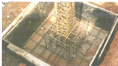
Figure 10 shows the formwork for pad footing.
