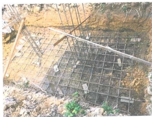
Figure 122 shows the installation of reinforcement.
