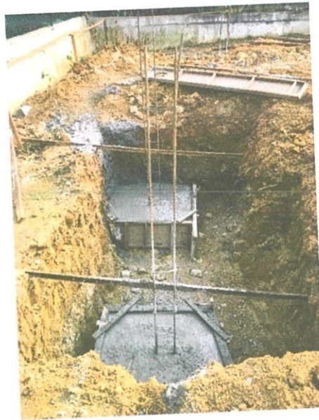
Figure 14 shows the process of curing.
