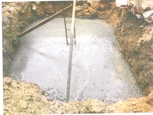
Figure 111 shows the process of lean concrete.
