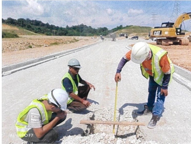
Figure 3.28: Excavate and Measure The Thickness of Crusher Run
