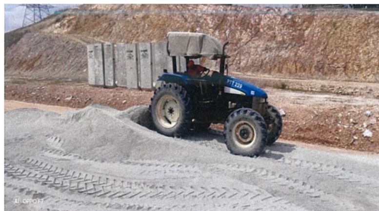
Figure 3.24 Back Pusher Spreading Granular
