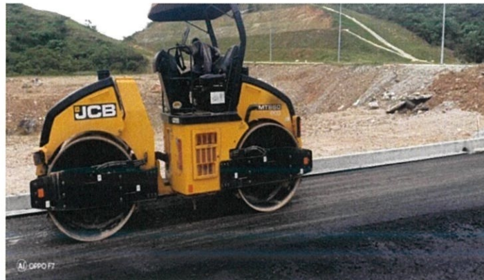
Figure 3.34: Tandem Roller Compacting Premix
