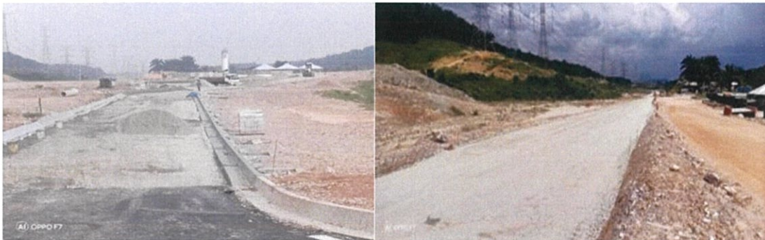
Figure 3.2: construction site 1 construction site 2
