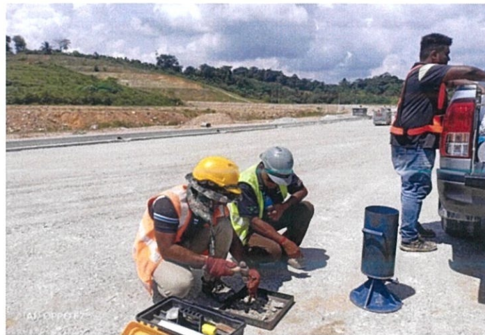
Figure 3.27: Field Density Test
