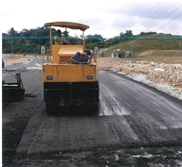
Figure 3.35: Pneumatic Tyre Roller Compact for Final Finishing
