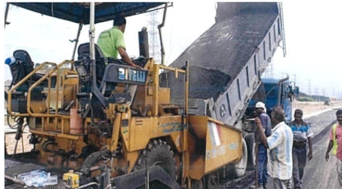
Figure 3.32: Fresh premix transfer to Paver Machine
