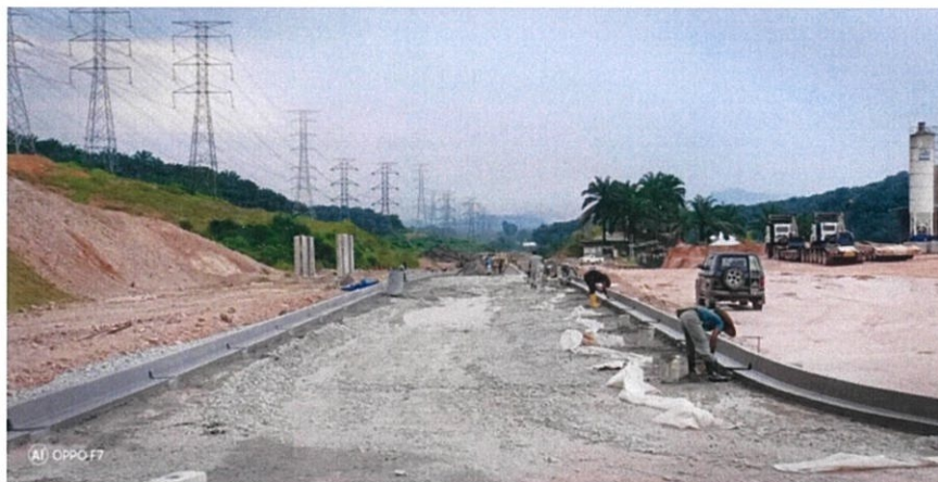
Figure 3.25: Spreader Crusher Run
