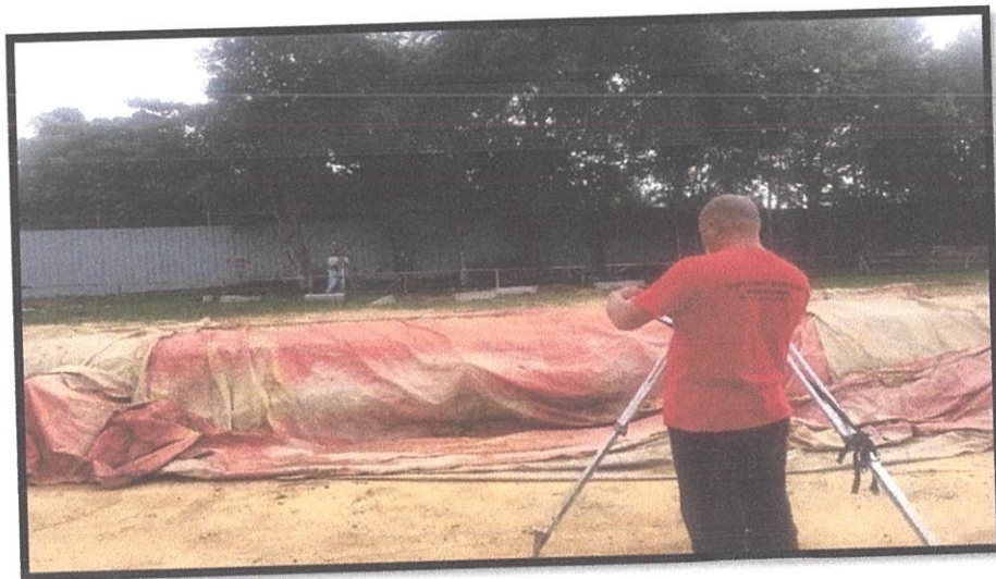
Figure 3.2.1: Surveyor survey the site
