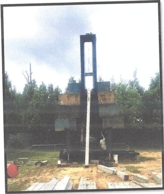
Figure 3.2.2: Pull pile using crane on board
