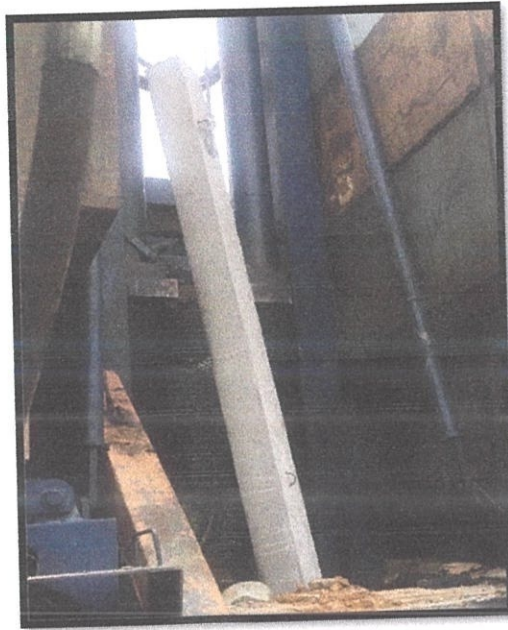
Figure 3.2.3: Insert the pile into the clamp
