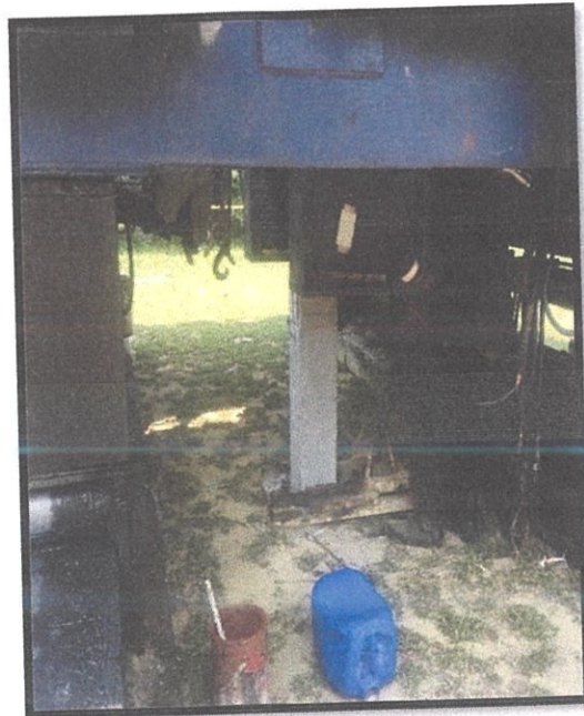
Figure 3.2.5: Press down the pile
