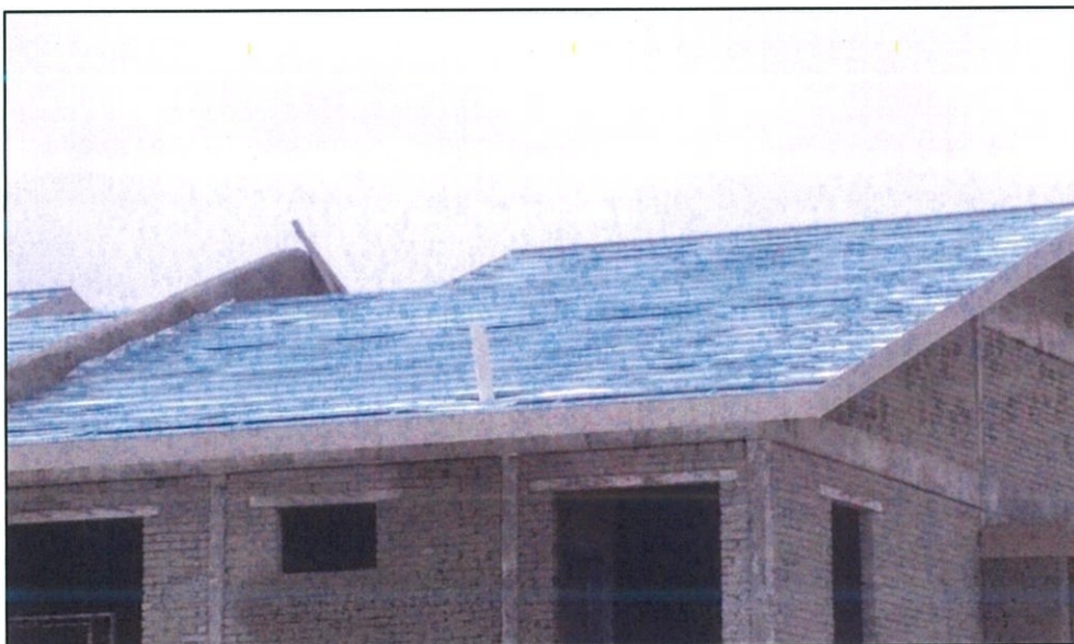
Figure 3.8: Foil paper and battens finished fixed
