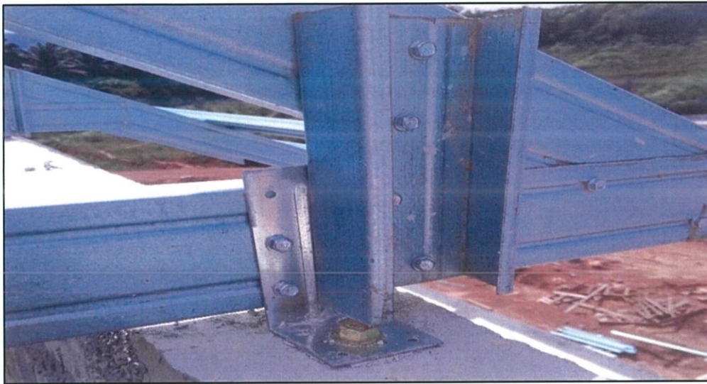
Figure 3.7: 'L' Bracket installed to the roof beam and truss
