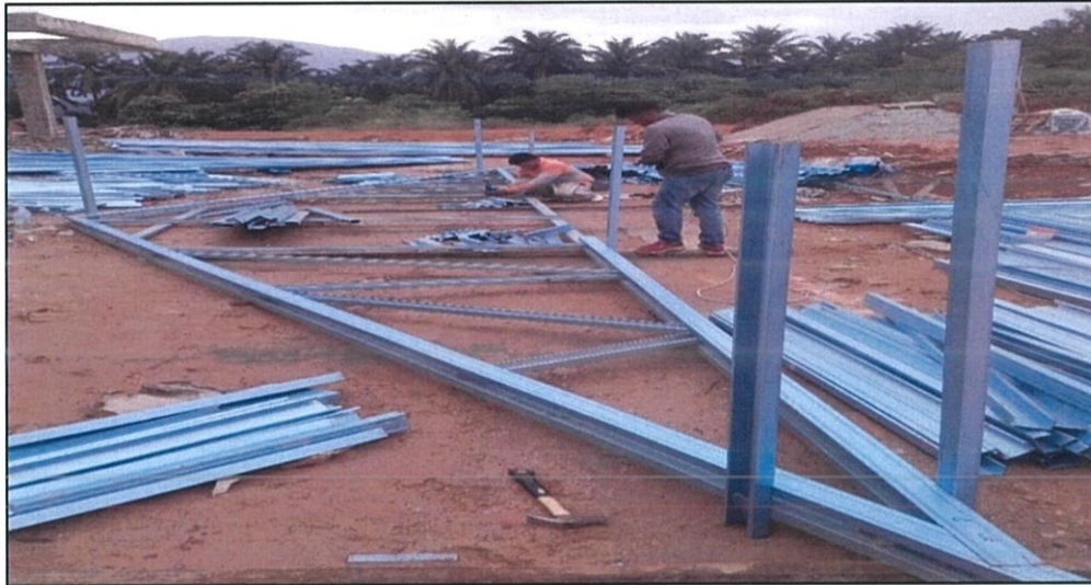
Figure 3.5: Workers are fasten the subsequent members
