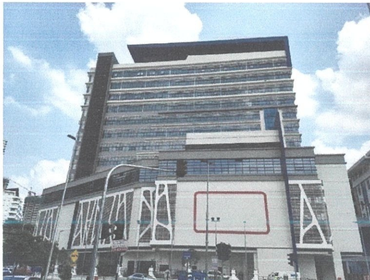
Figure 3.3 View of the building
