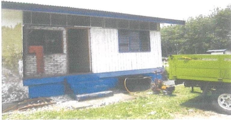
Figure 3.1: Building maintenance at Balai Polis Banggol Judah, Machang, Kelantan
