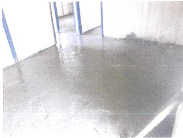
Figure 3.2: Laying of new floor
