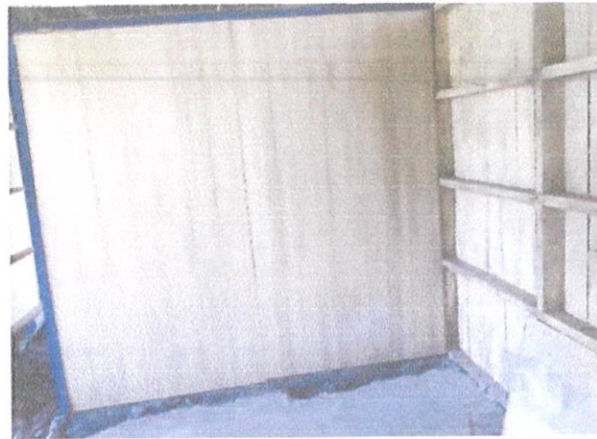
Figure 3.3: Erection of new Wall
