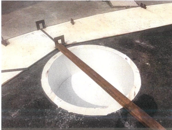
Figure 3.2: Arrangement of sump tank
