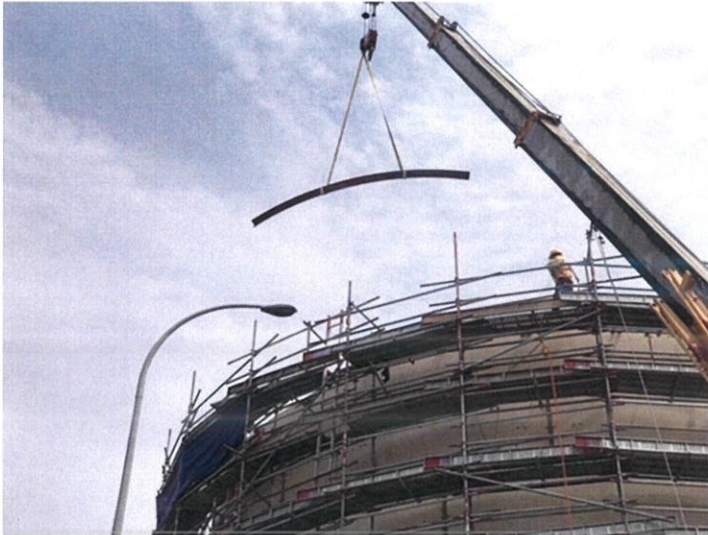
Figure 3.8: Installing the roof ring
