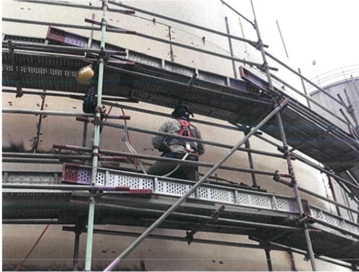
Figure 3.6: Welding the outer of shell plate
