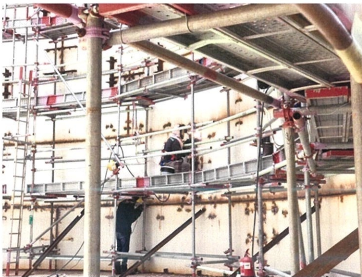
Figure 3.7: Welding and grinding the inner of shell plate
