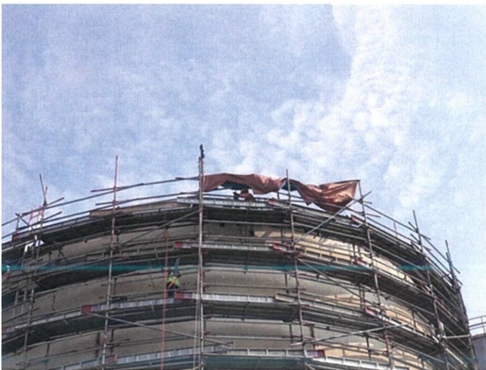
Figure 3.9: Welding the roof ring
