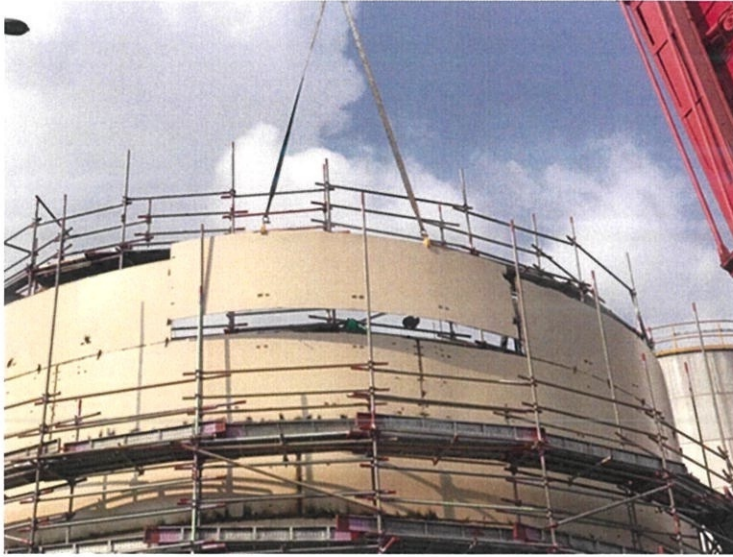
Figure 3.4: Installing the shell plate level by level
