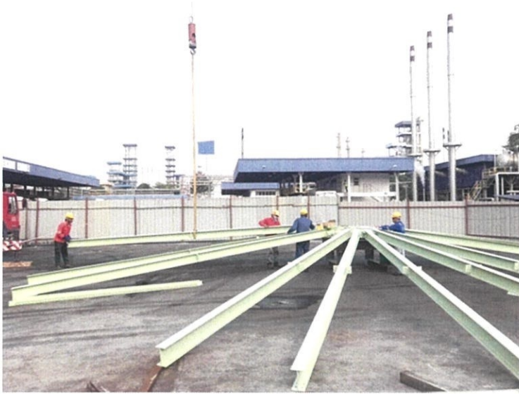
Figure 3.10: Arranging and installing the roof structures
