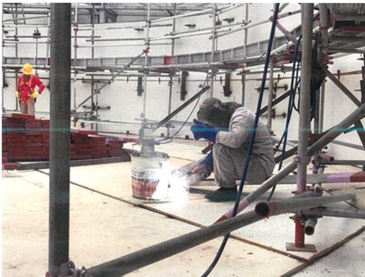
Figure 3.5: Welding the bottom plate
