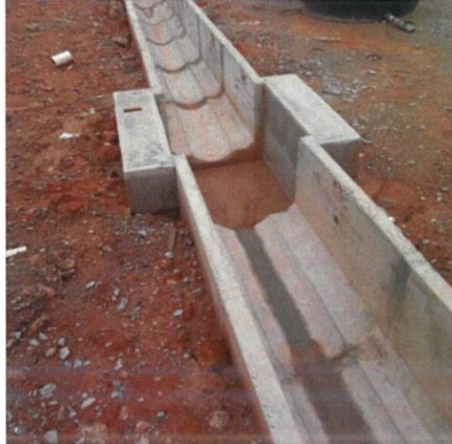
Figure 3.11 : Installation of pre-cast U drain completed
