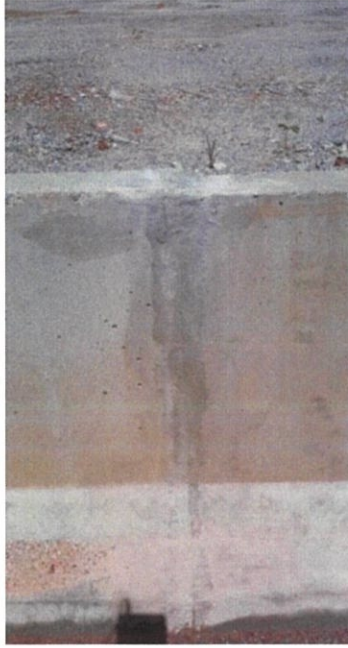
Figure 3.9 : Closer look of gap filled with mortar joint
