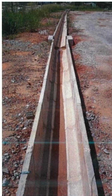
Figure 3.10 : Mortar joint in all drains on external sides
