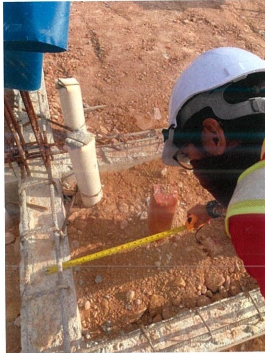
Figure 25 Inspect Distance of Pipes
