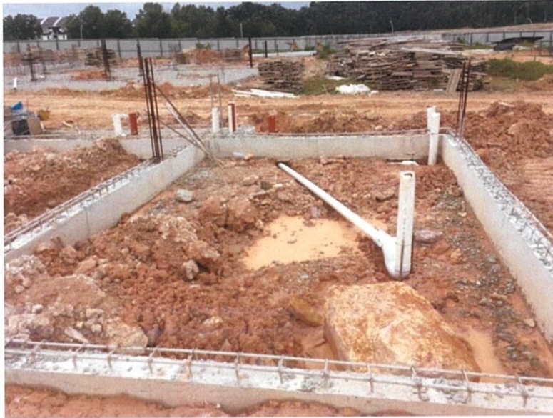
Figure 19 Floor Trap Installed
