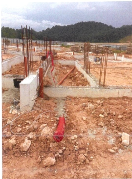
Figure 22 Corrugated Electrical Pipe Installed
