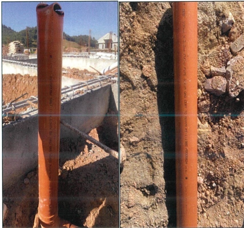
Figure 10 Water Closet Pipe
