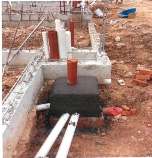
Figure 21 Gully Trap
