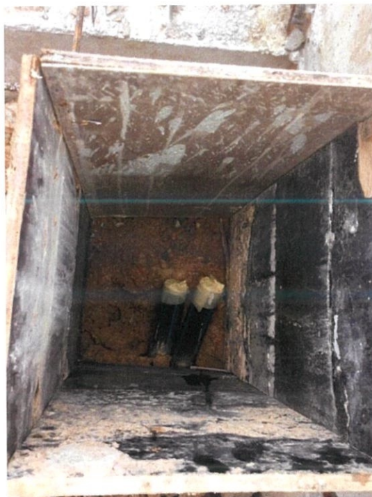
Figure 24 Telephone Pipe Installed
