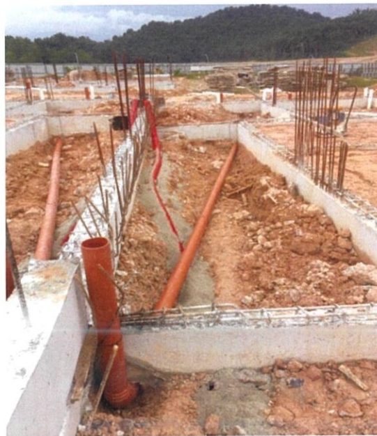
Figure 20 Water Closet Installed
