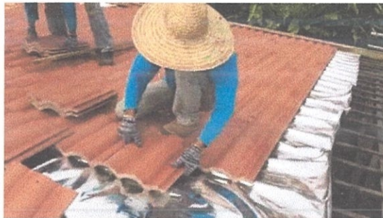
Figure 3.18: Rafter install roof tiles
