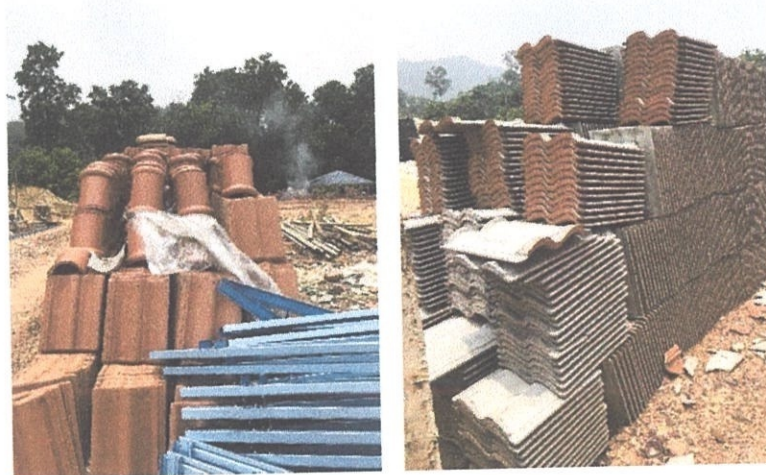
Figure 3.13: Material on Site
