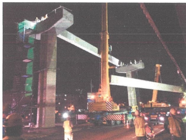
Second u-beam launching for the second night
