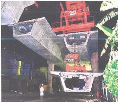
Figure 3.3 & 3.4: Example of box girders
