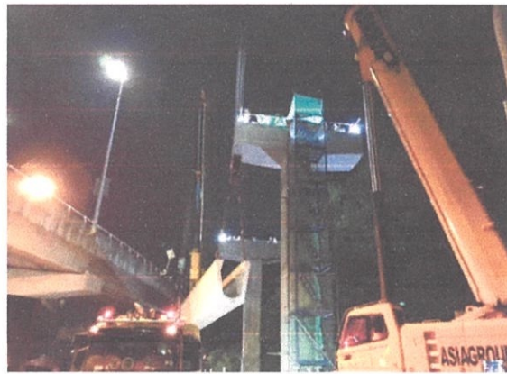
The first u-beam launching
