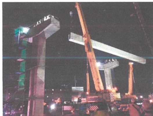
Photo 3.1: Lifting of beam
