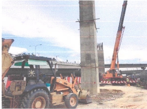
Excavation and laying crusher run to make good access
