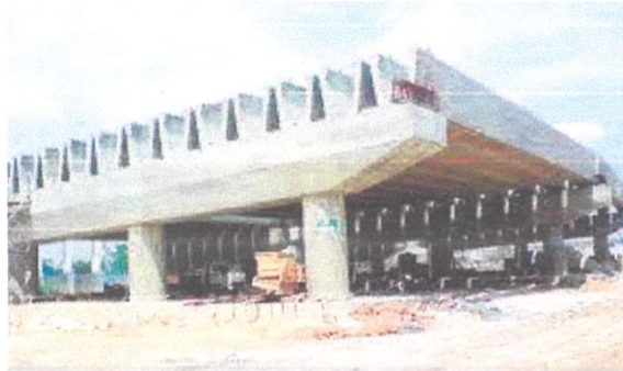
Figure 3.11: Example of u-beam on piers
