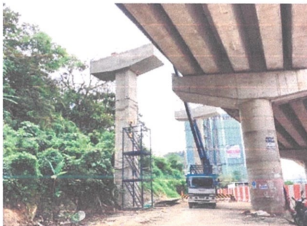
Assembling access at the side of the pier
