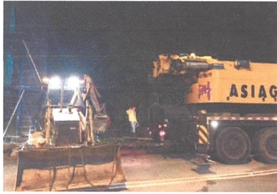
Parking of crane before the beam launching
