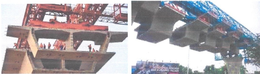
Figure 3.8 & 3.9: Example of box girders
