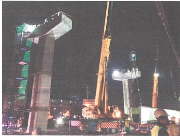
The first u-beam launching for the second night at different piers
