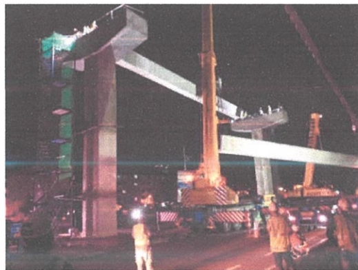
Photo 3.2: Lifting of second beam
