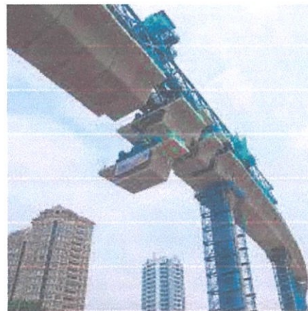
Figure 3.3 & 3.4: Example of box girders
